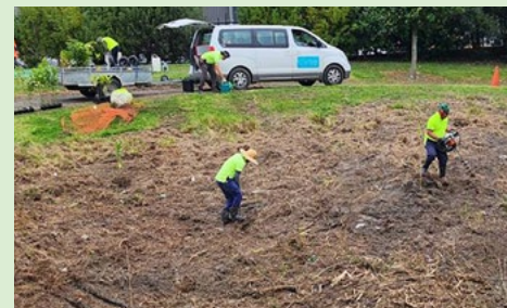
Banks along the coastal margin were cleared of thick tree weed cover before planting could start. Tall privet and wattle trees, mature woolly nightshade, gorse bushes, pampas clumps, blackberry vines, bone seed and many other species have taken over the banks and created an environment that is hostile to native animal and plant life.
